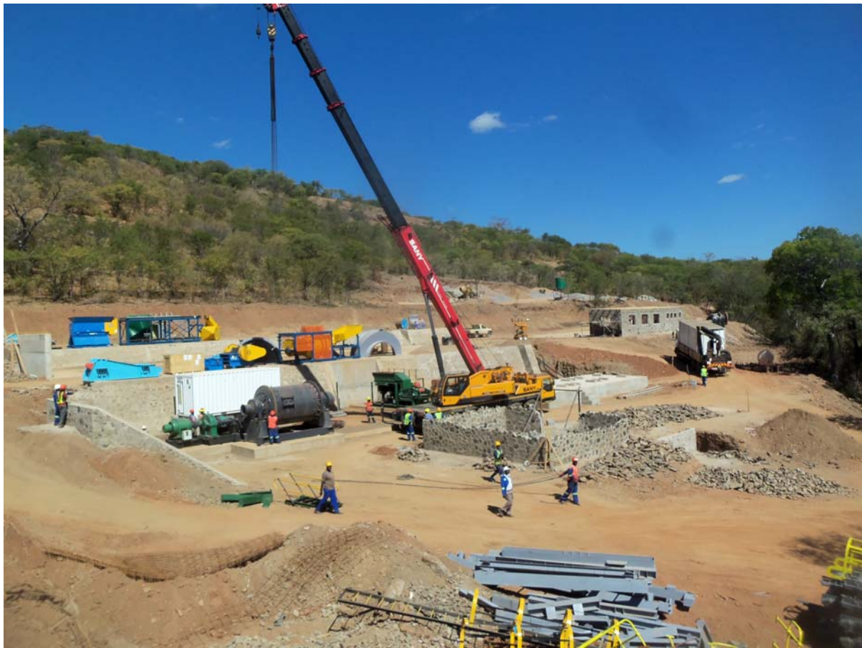
Offloading of plant completed 24 May 2015
