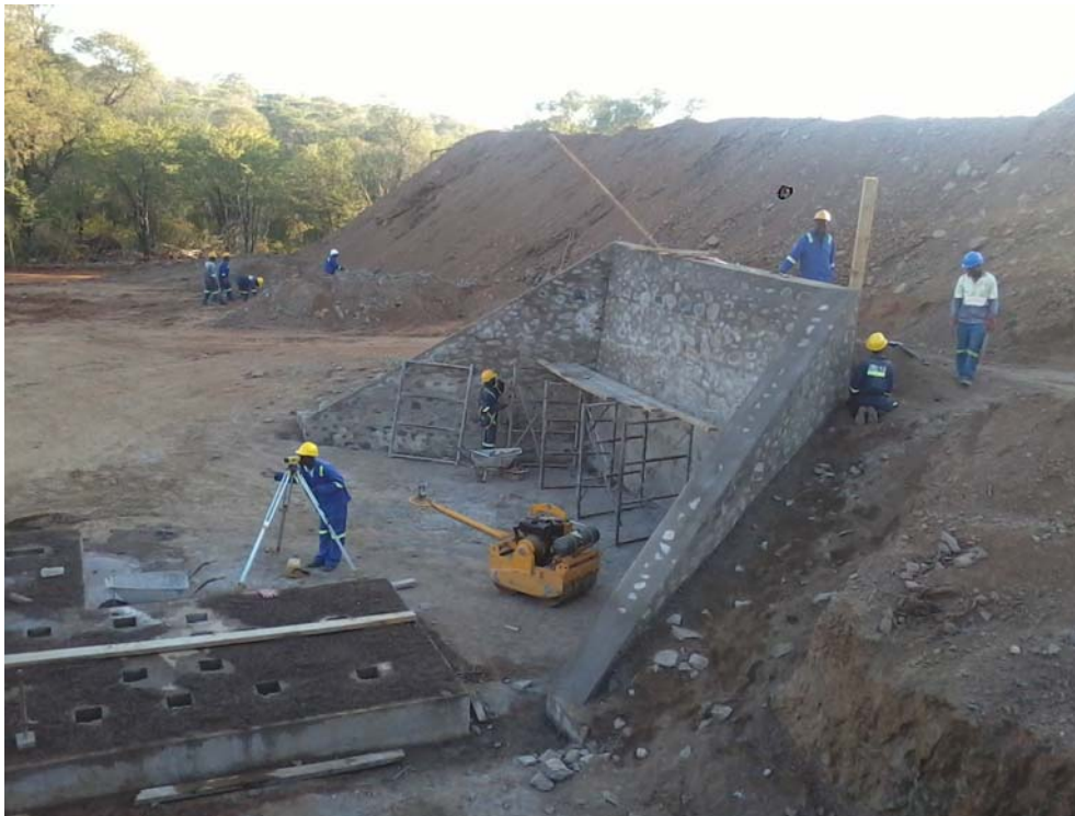
Retaining wall for Rod recharger
