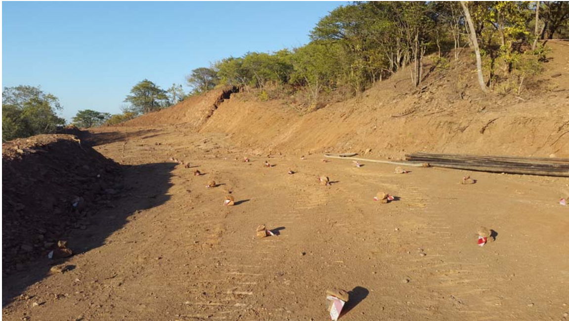
Blast block pegged out on 965 level
